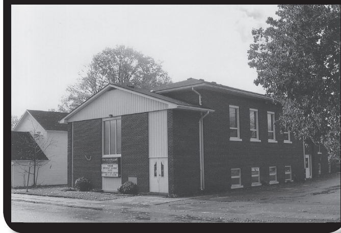
"New" Wingham PRC building
