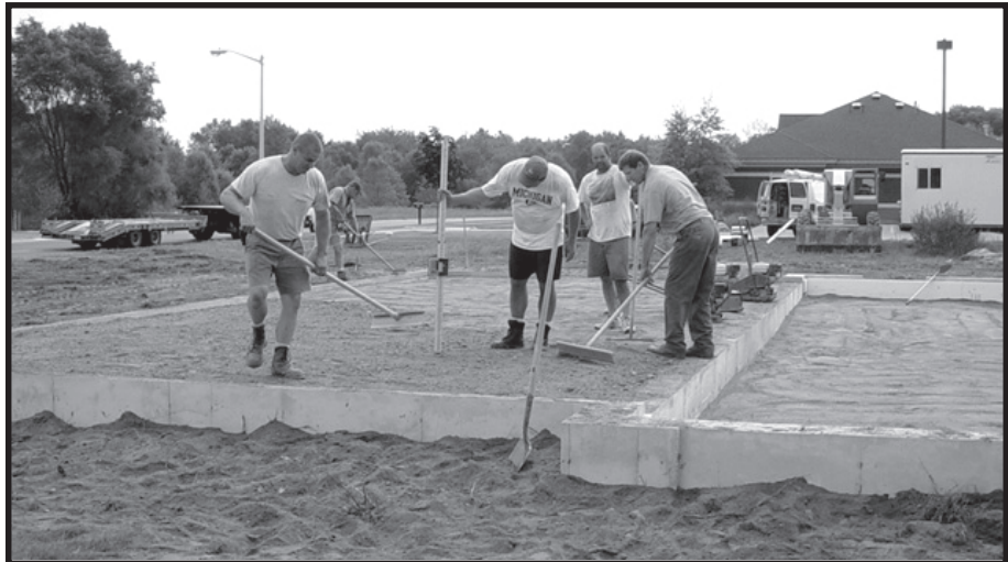
Standing in the future office area, volunteers work to backfill and grade in preparation for concrete. The office area will overlook Georgetown Center Drive near 20 th Avenue and Baldwin in Jenison.
