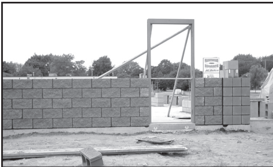
As the block is laid, the service door frame to the shipping area is set in place. The 16' x 24' shipping area will hold a limited inventory of each of our books, from which we can easily fill orders.
