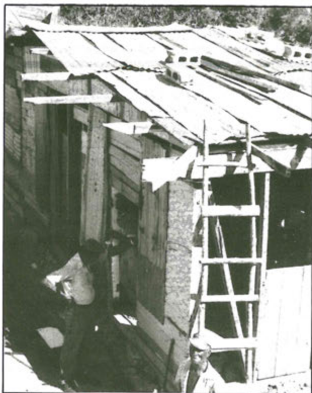
Many roofs were lost in the storm. Here Deacon Carr, in Dias, has replaced the pieces of zinc and, for lack of nails, simply weighted them down with cement blocks.
