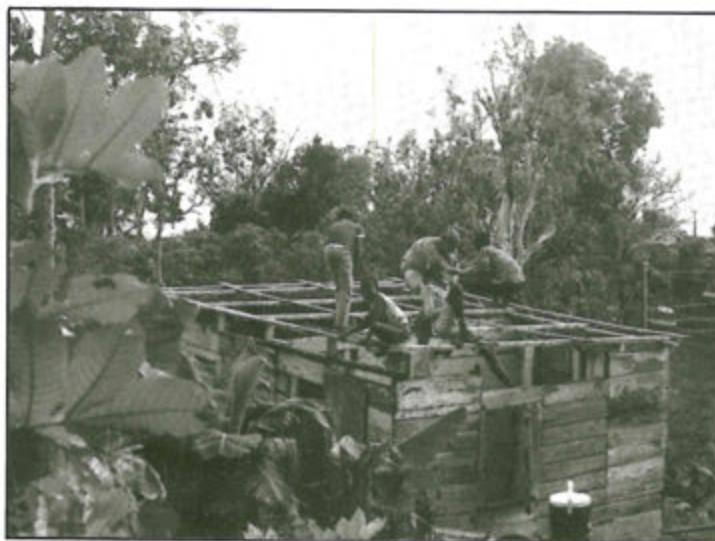
The carpenters took zinc nails with them from the States. Here they replace a roof on a house in Cave Mountain (with the help of local talent).
